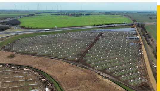
PV-project "Kreuz Uckermark" by ENERTRAG during the construction phase
